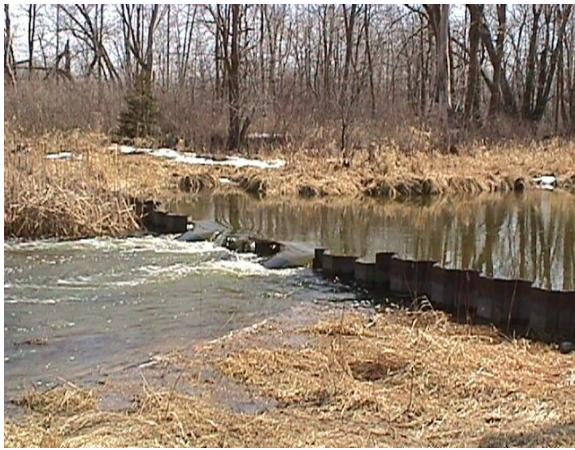
Sheet Piling Weir with 2 adjustable stoplog bays
