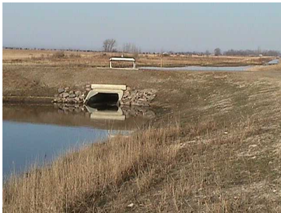
Site #1 Principal Outlet Structure
