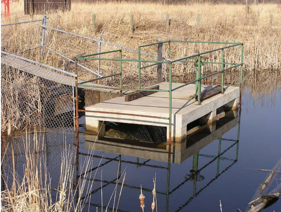
Outlet Control Structure Outlets to Marshall County Ditch #200
