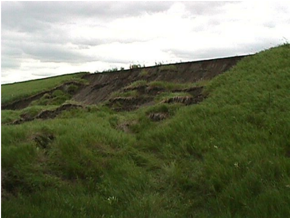
Slope Failure
