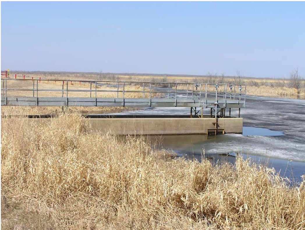
South Pool Principal Outlet Structure Outlets to Judicial Ditch #11 (Mud River)
