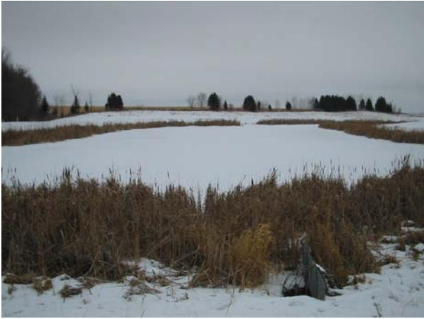
Thibert Dam, Red Lake County
