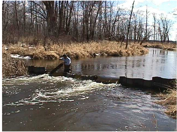
Removing stoplogs to manage lake level
