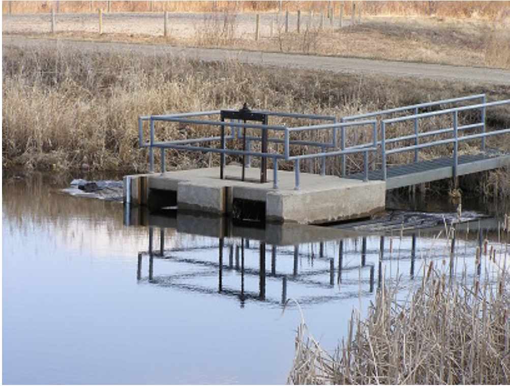
Principal Outlet Structure
