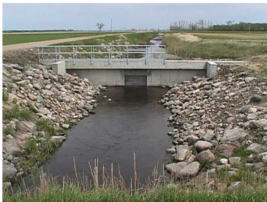
Parnell Impoundment South Outlet Control Structure Judicial Ditch #60 Weir Operable Gate
