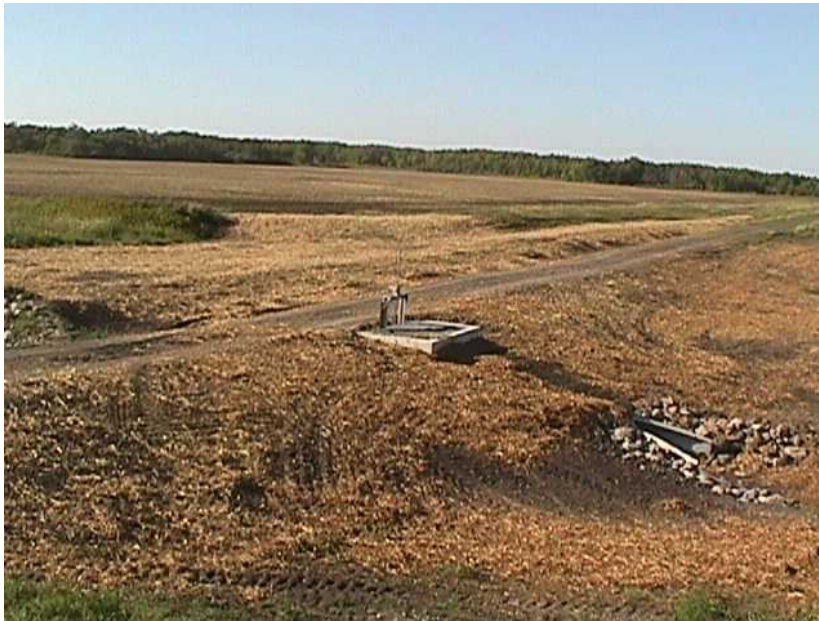
North Parnell Storage Site Outlet Control Structure
