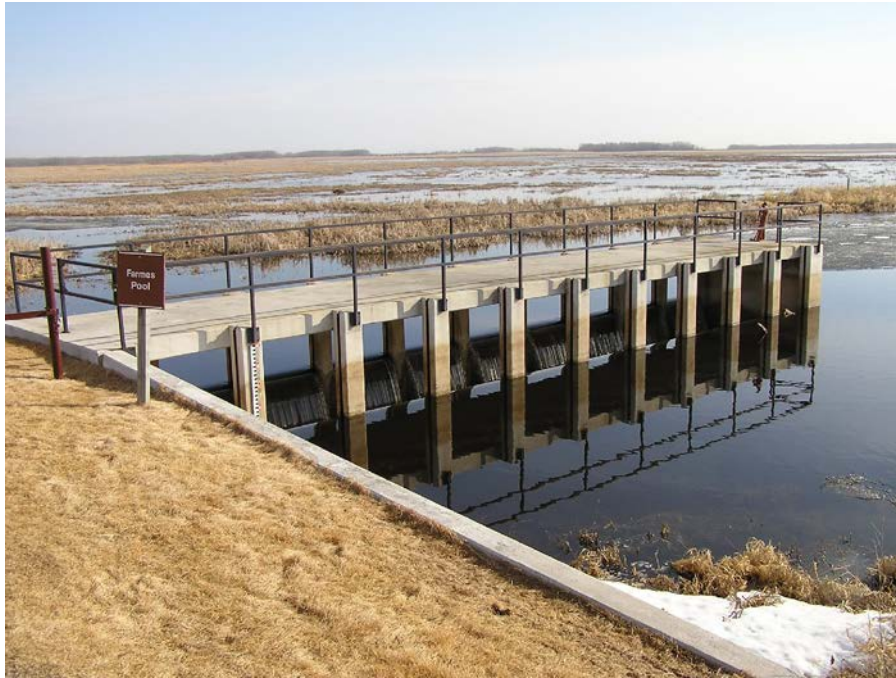
Principal Outlet Structure Outlets to Marshall County Ditch #200 approximately 2 miles upstream of the Thief River
