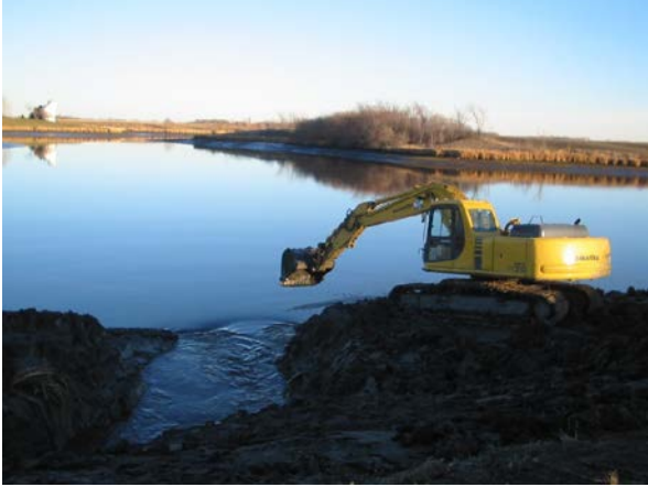
Excavation for Pool Drawdown
